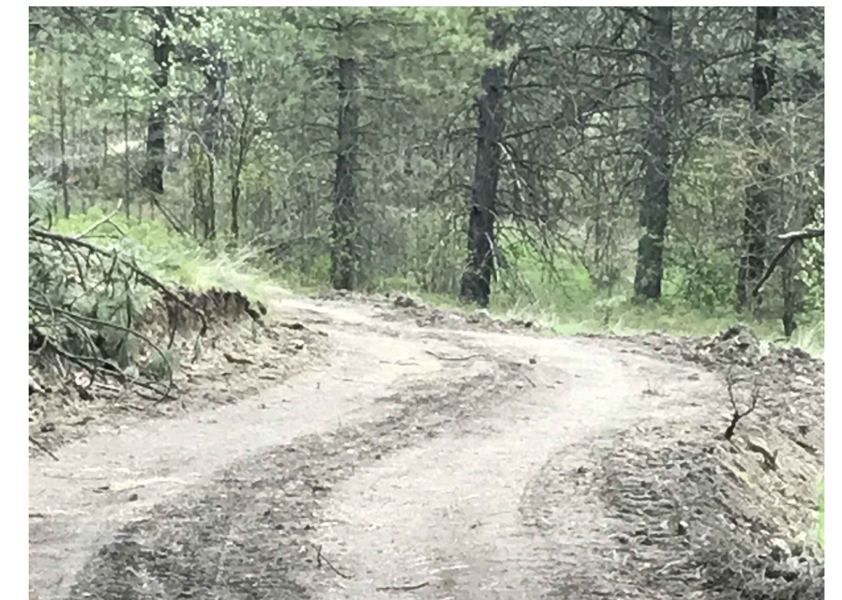
5. MODERATE ROAD CUT/FILL
