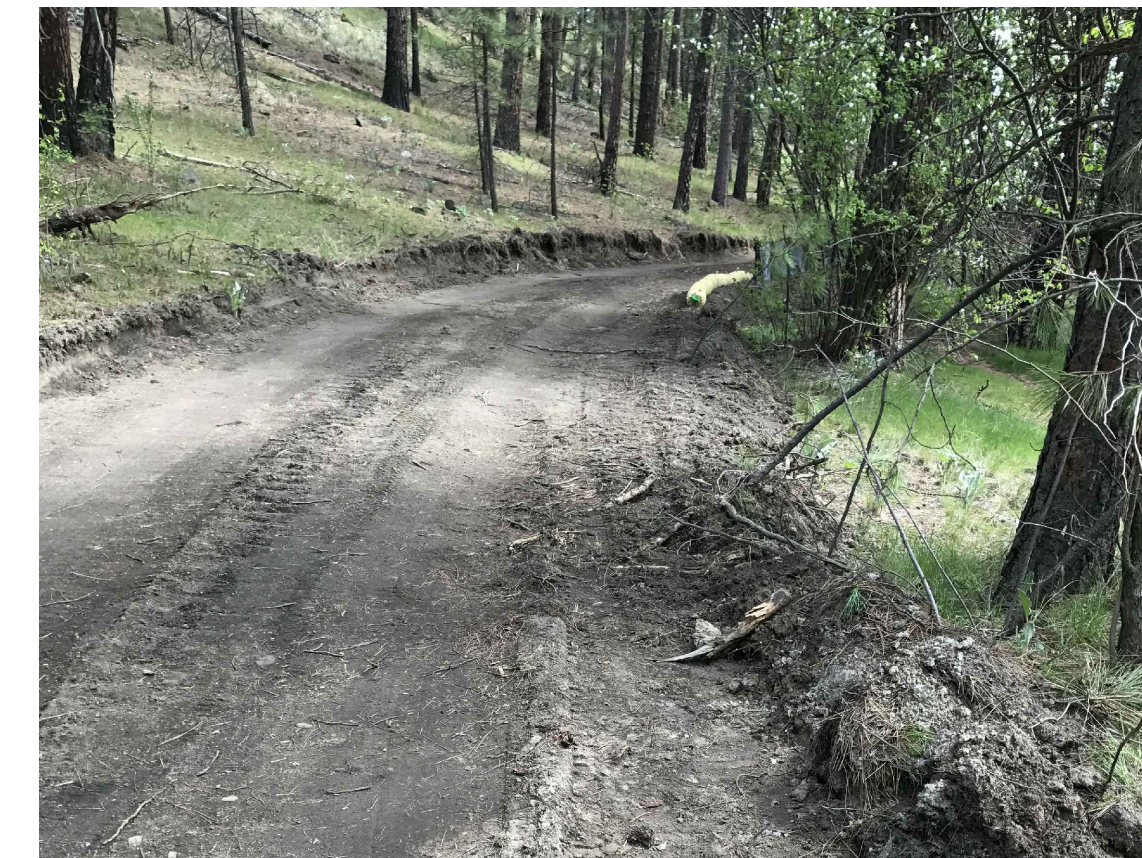
3. MODERATE ROAD CUT/FILL
