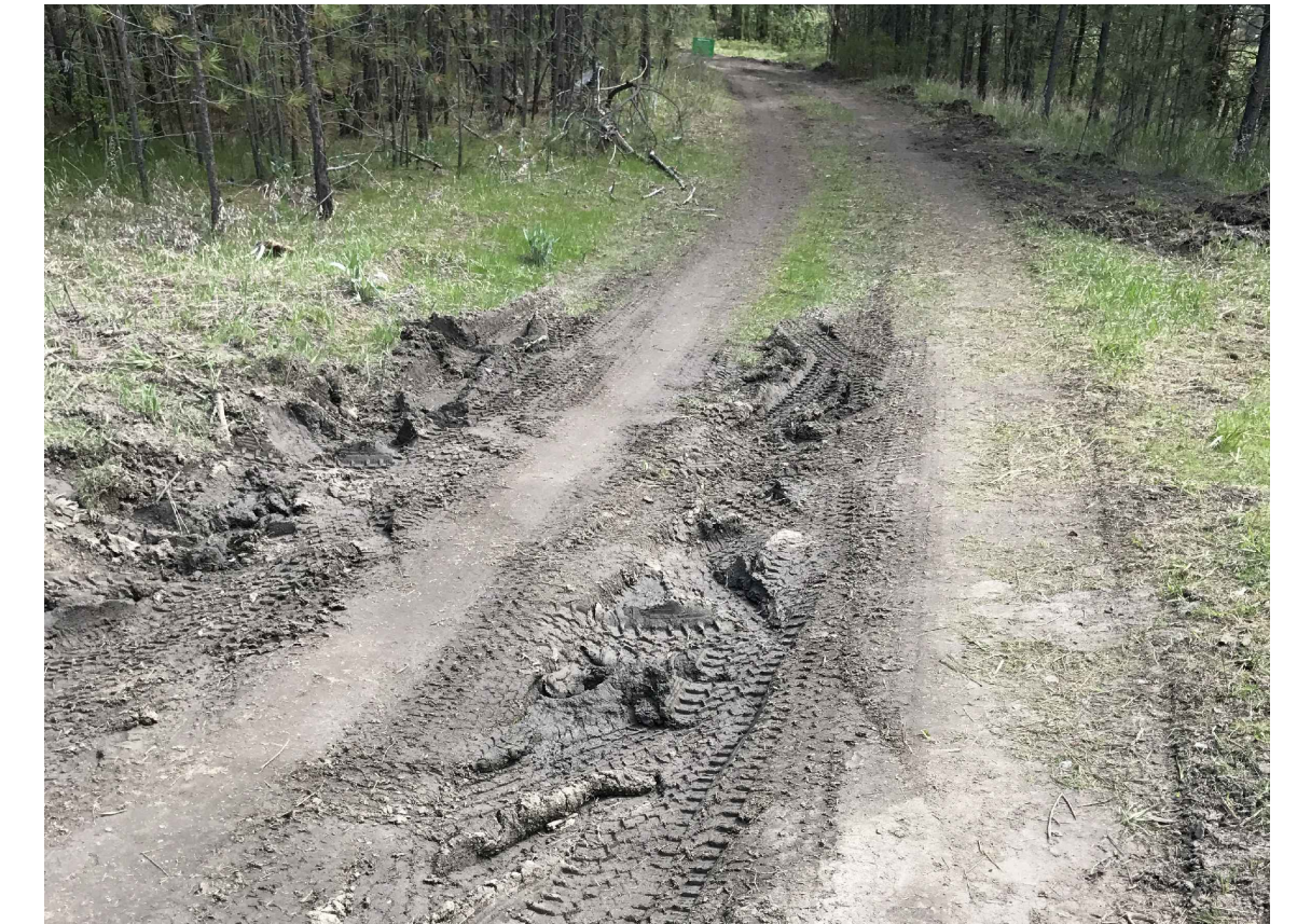
2. BEGINNING OF NEW BLUFF ROAD
