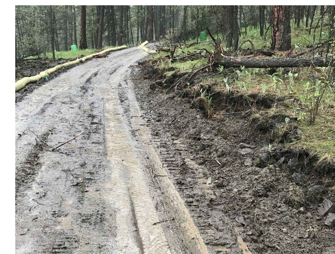
8. MODERATE ROAD CUT/FILL
