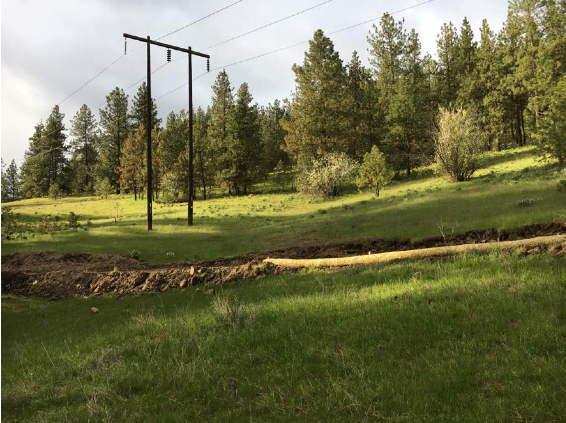
Photo 4. Transmission line right-of-way with grass and forb community and open space
