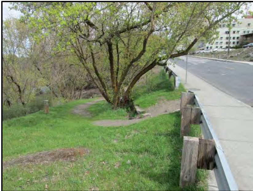
Photo 16: Looking easterly at the area where the proposed trail alignment would connect to Main Avenue, along the northern sidewalk.
