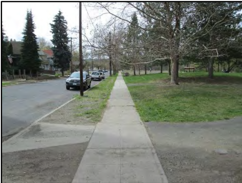
Photo 12: Looking westerly along the proposed trail alignment (on the north side of Water Avenue). This photo was taken directly underneath the Maple Street Bridge. Ornamental trees in this area would be retained.
